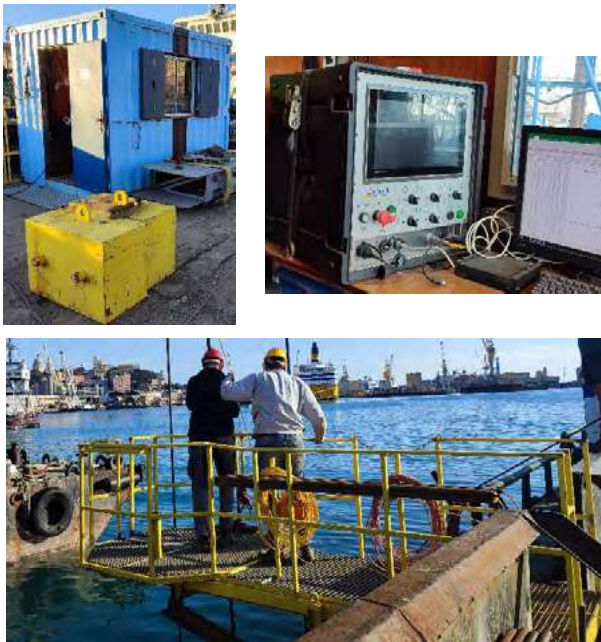
Figure 5. Office Container, Manta control unit and cantilever
