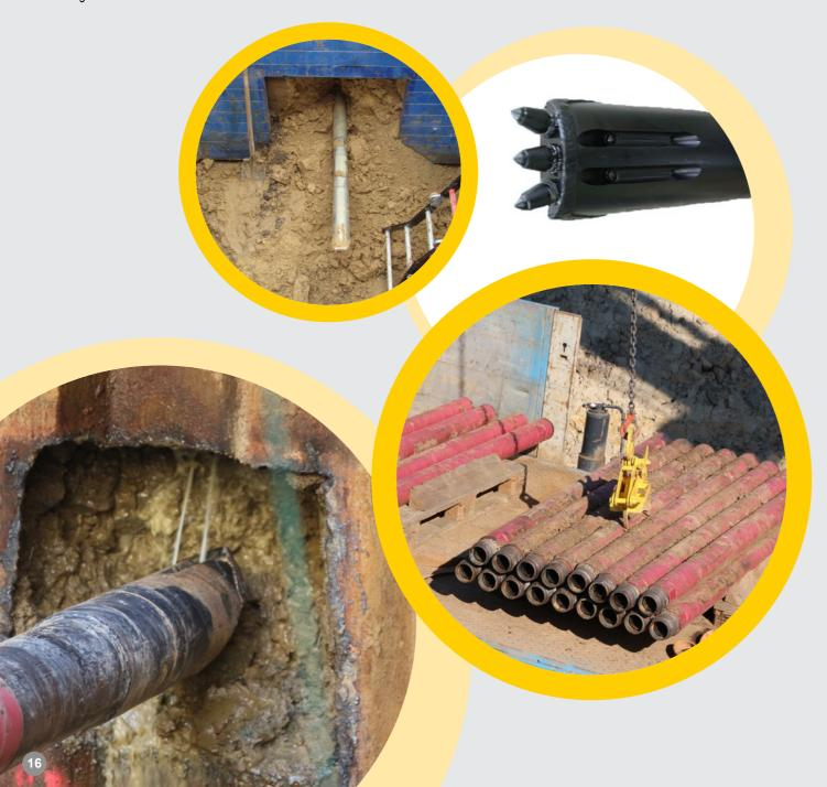
The pipe controls allow for the laying of steel pipes with diameters between 406 and 1.400 mm in any subsoil, from cohesive soils and unconsolidated rock, right through to solid rock, in one operation. The horizontal (RS) and the horizontal and vertical (RS-HV) versions can be precisely controlled by means of articulated pipe sections that can be adjusted hydraulically.
